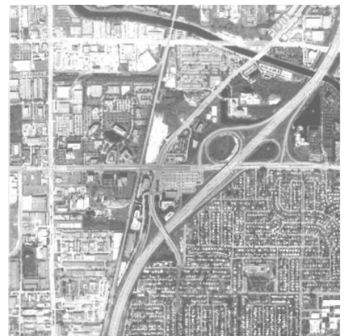
Cypress Creek Road and Andrews Avenue in 1963 (top), 1976 just after initial construction of I-95 (middle), and 1995 after the widening project (bottom).
